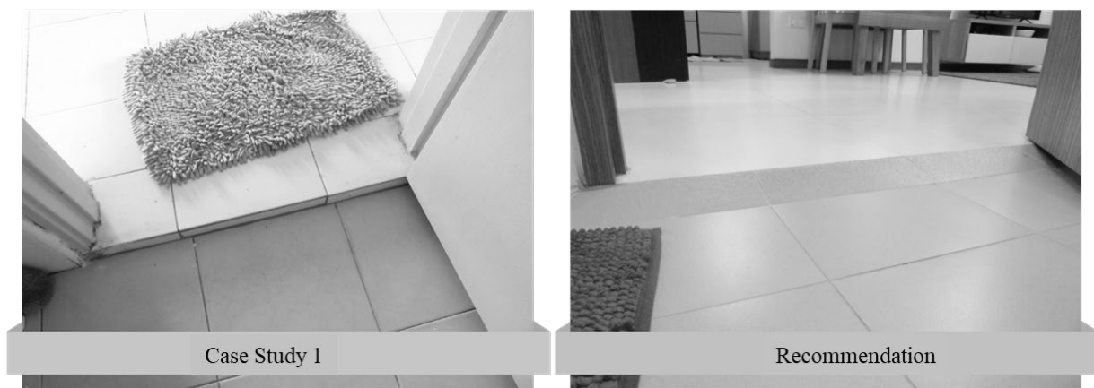
Fig. 7. Case study 1 internal threshold and the recommended solution to improve circulation
