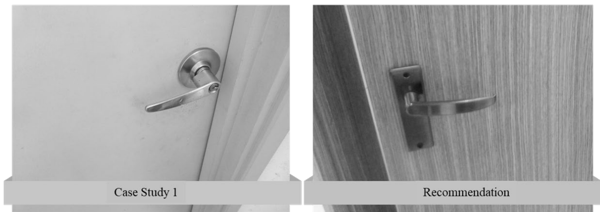
Fig. 11. A U-shaped door handles recommendation
